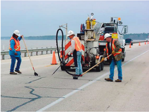
Crack Sealing
