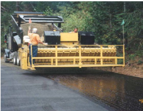
Surface Treatment (Chip Seal)
