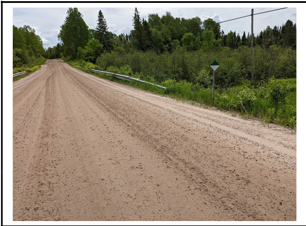
Photo 9 Gravel approach wearing surface
