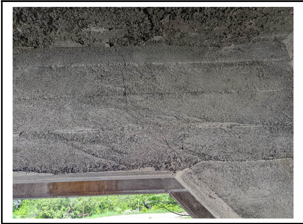
Photo 13 Narrow crack on girder
