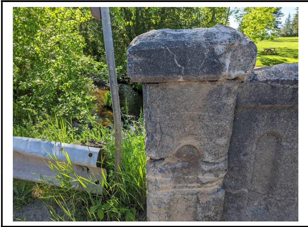
Photo 9 Substandard connection at northwest approach barrier (Typical)
