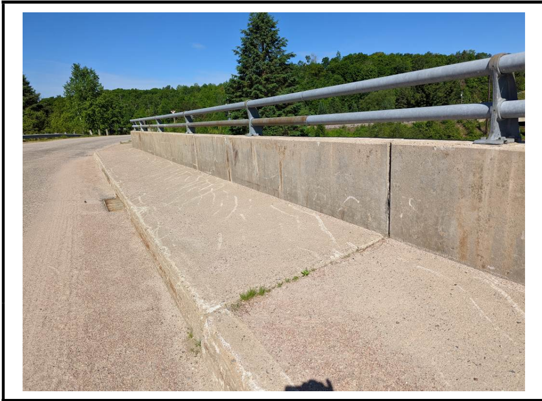
Photo 11 Narrow map cracks with efflorescence and stains with spall on parapet wall
