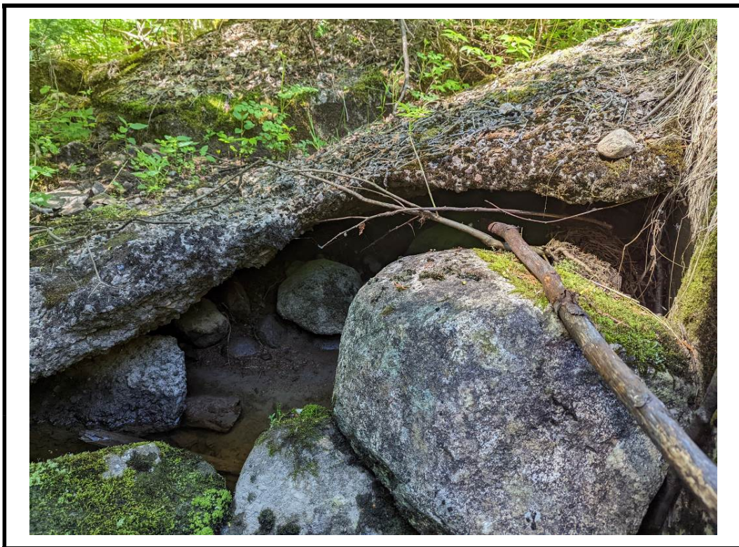
Photo 18 Concrete slope protection at southwest corner failed
