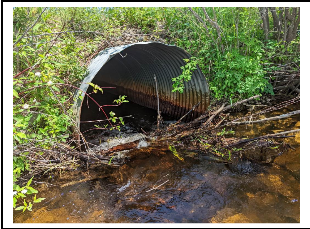
Photo 9 Beaver dam observed at south end of east barrel
