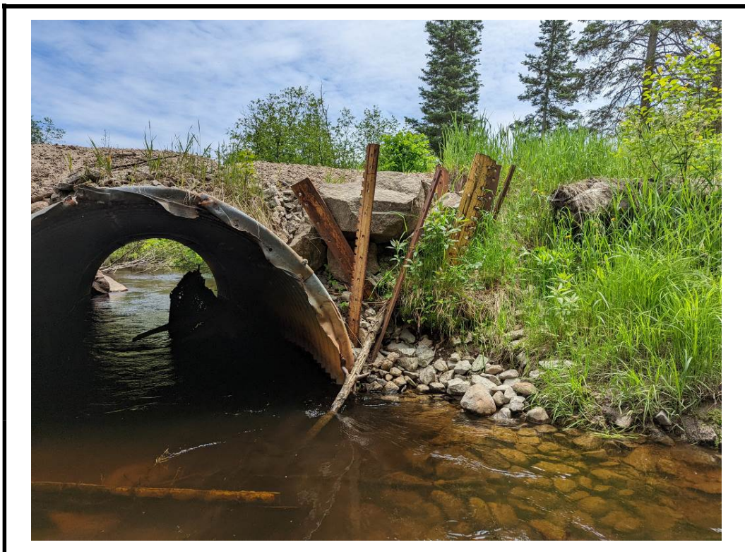
Photo 8 Dents noted at west end of barrel
