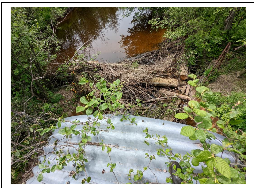
Photo 10 Obstruction at west end of north culvert.
