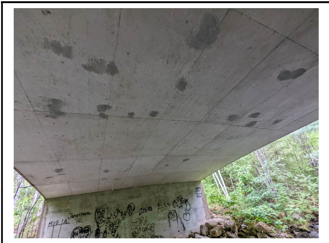
Photo 10 Typical deck soffit with previous concrete repairs
