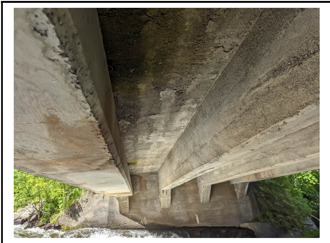
Photo 12 Light scaling on interior deck soffit
