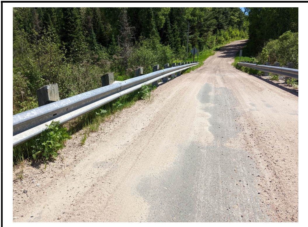
Photo 8 Longitudinal grooves on structure wearing surface
