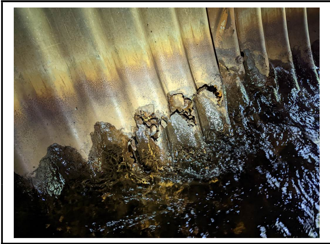
Photo 11 Localized perforation at bottom of barrel, near north end of barrel
