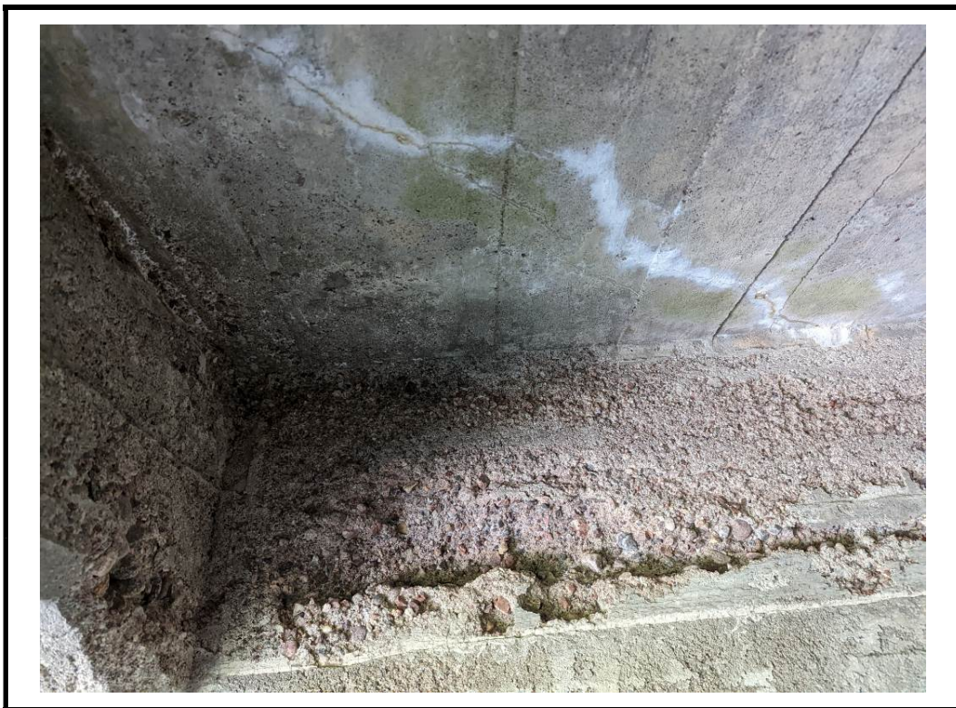
Photo 16 Severe scaling on ballast wall and cracks with efflorescence noted on deck soffit
