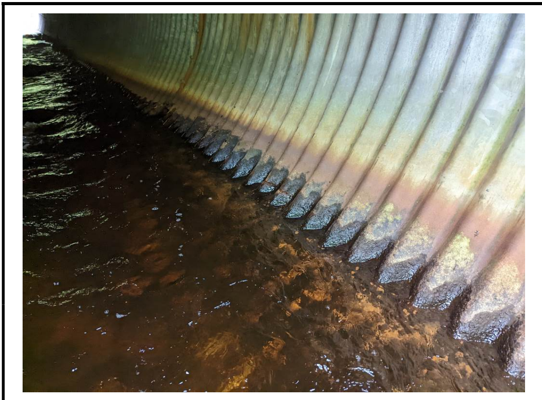
Photo 8 Moderate corrosion noted along bottom of barrel
