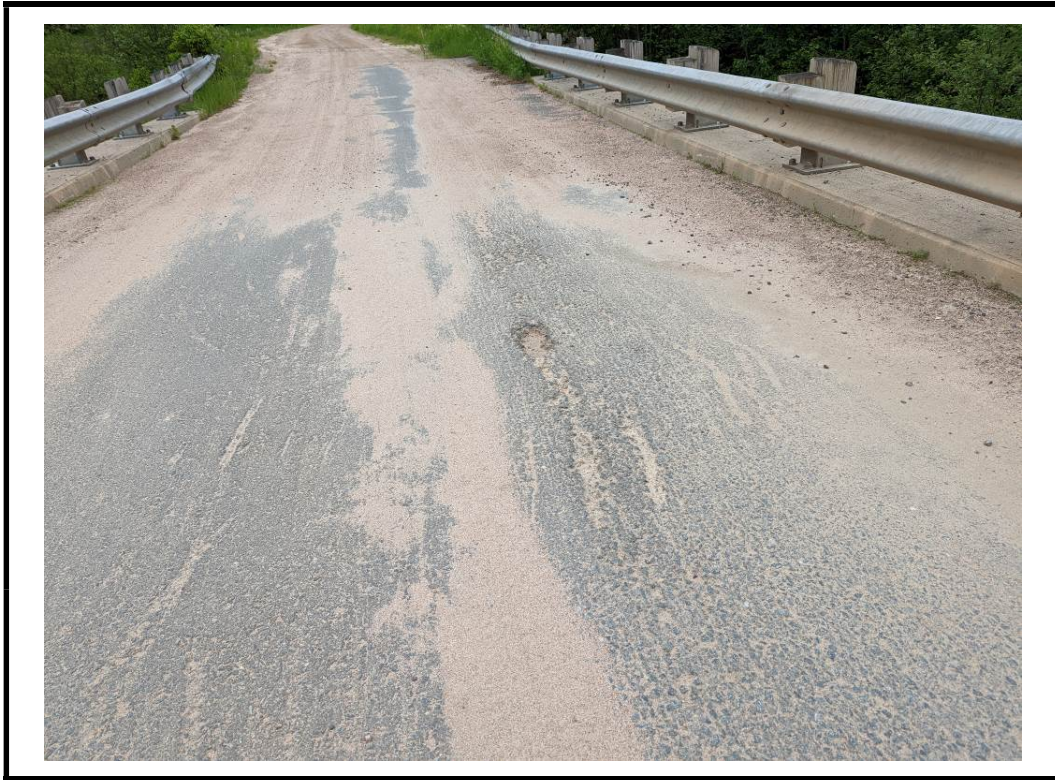
Photo 11 Minor scaling and small gouges noted in middle of deck wearing surface
