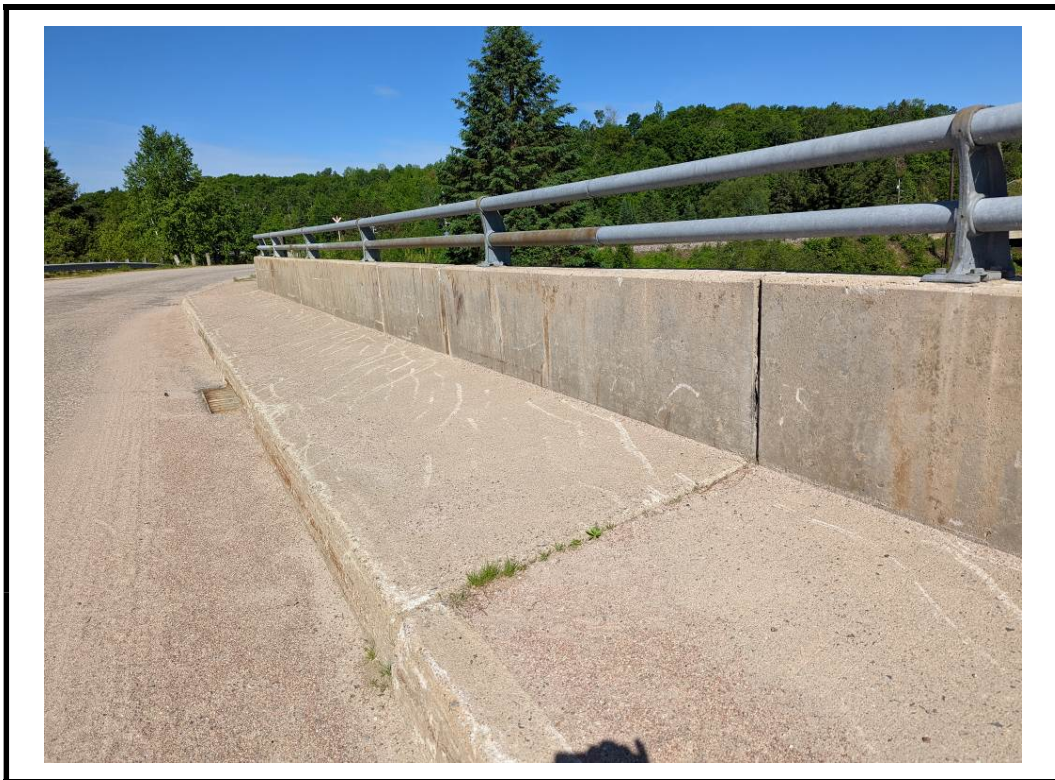
Photo 12 Narrow map cracks with efflorescence and stains with spall on parapet wall
