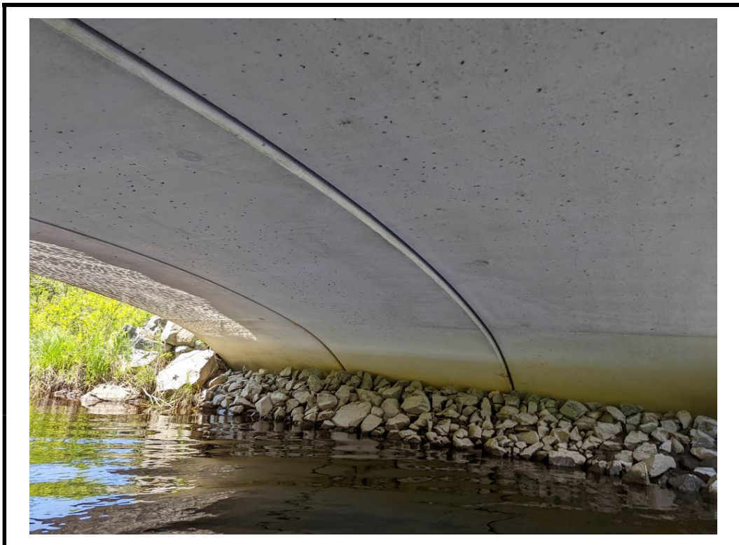
Photo 12 Bug holes noted throughout barrel soffit
