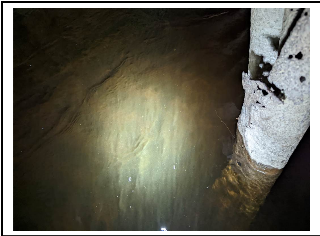
Photo 11 Severe perforation noted at and below waterline
