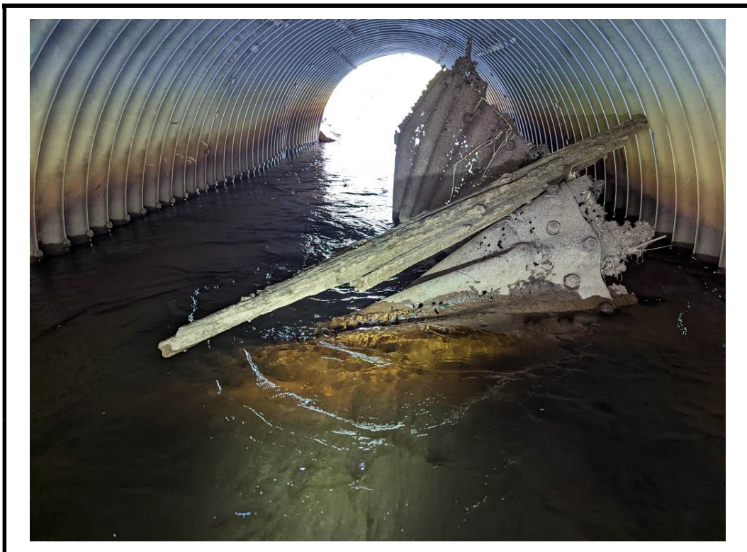
Photo 12 Damaged section of CSP in barrel, does not appear to be from this structure
