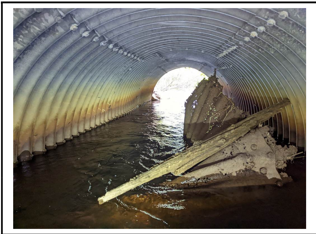
Photo 10 Efflorescence noted at seams and along boltline
