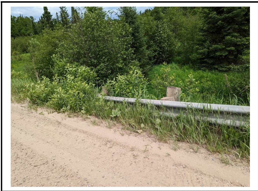
Photo 8 Substandard buried end treatment at approach barrier
