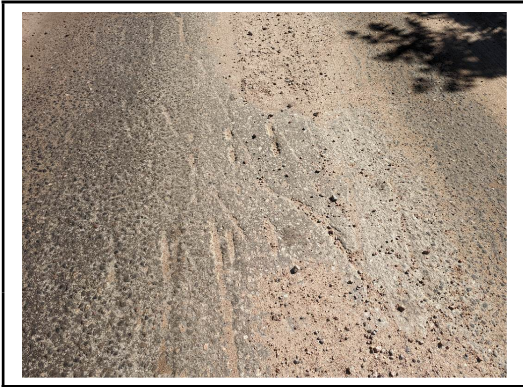
Photo 7 Moderate scaling, tire rutting and gravel accumulation in approach wearing surface (Typical)
