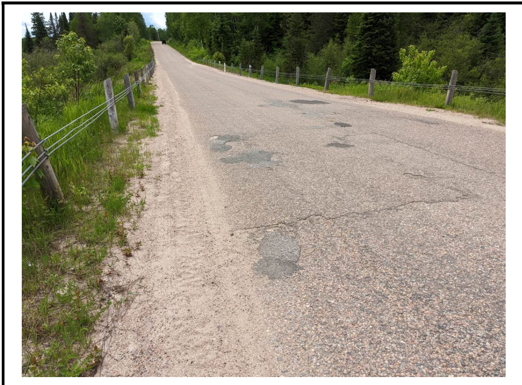
Photo 8 Moderate ravelling, patched potholes noted in east approach wearing surface
