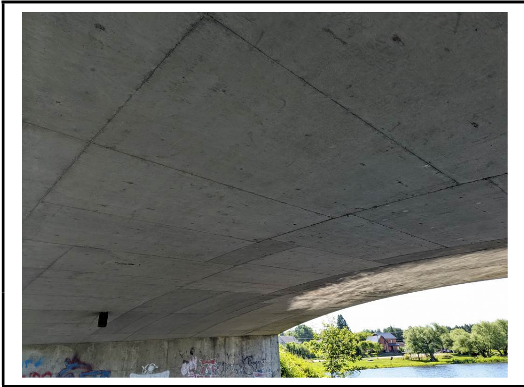
Photo 15 Typical deck soffit
