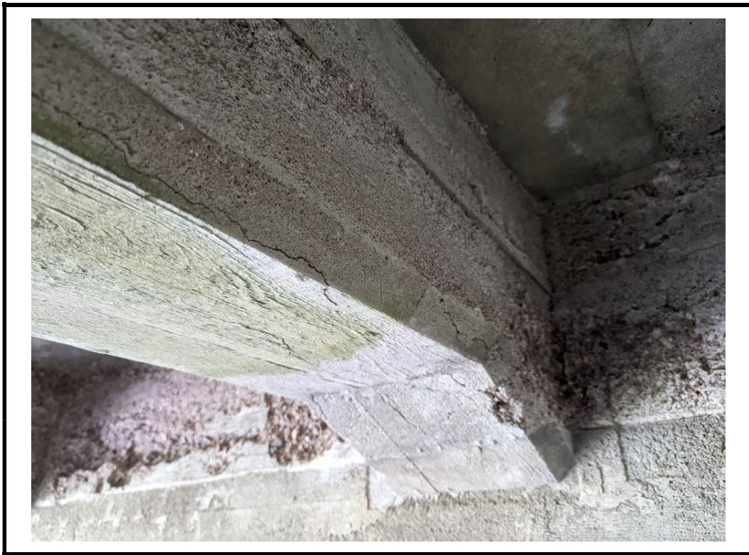
Photo 17 Spall and longitudinal cracks noted on girders
