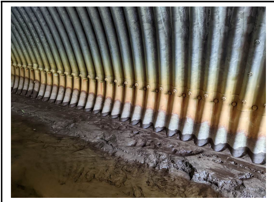
Photo 8 Light to localized moderate corrosion noted at and below waterline
