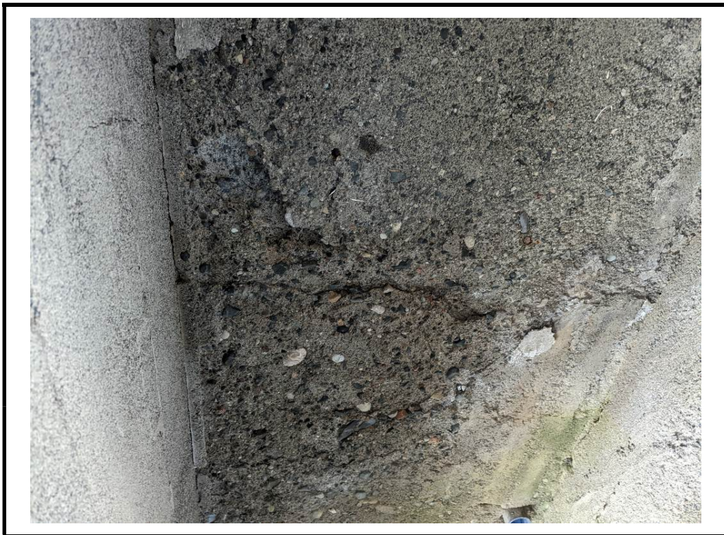
Photo 14 Moderate to severe scaling, narrow cracks and delamination noted on deck soffit
