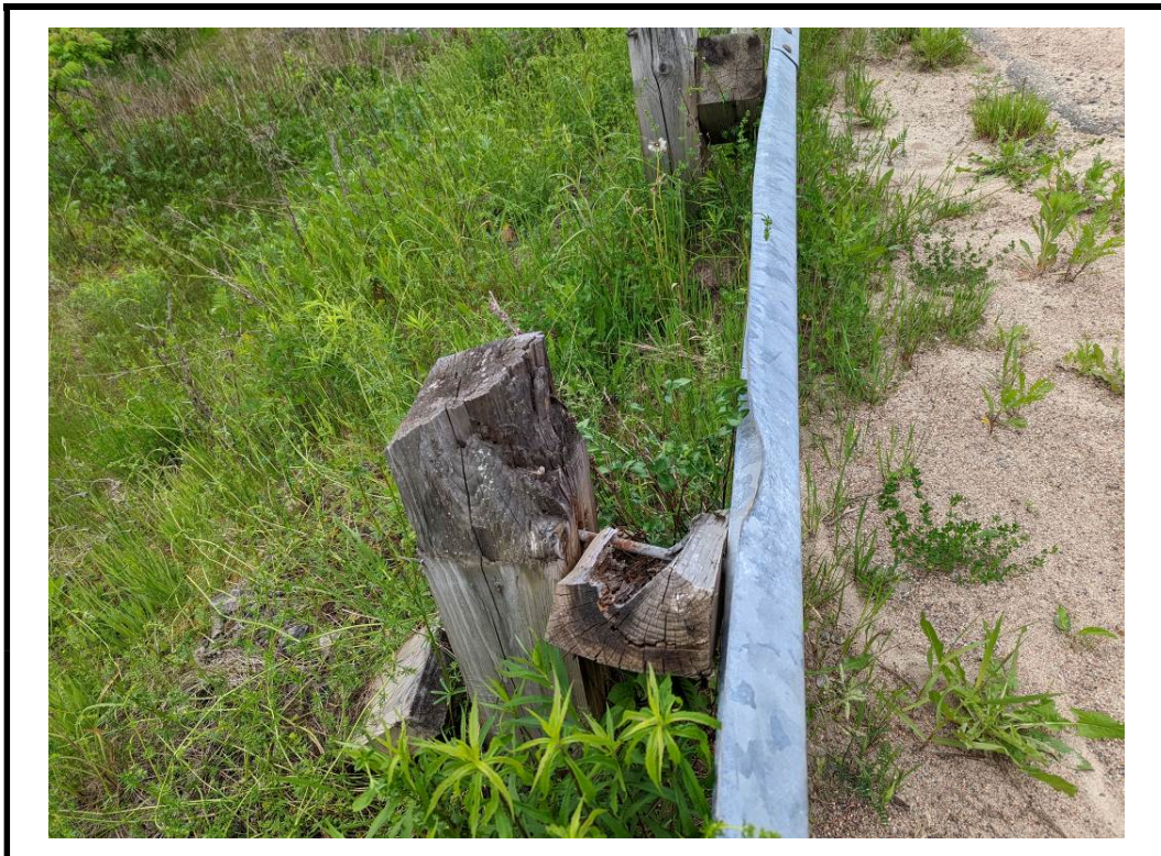
Photo 8 Checks and splits on barrier post with damaged and rotated spacer block
