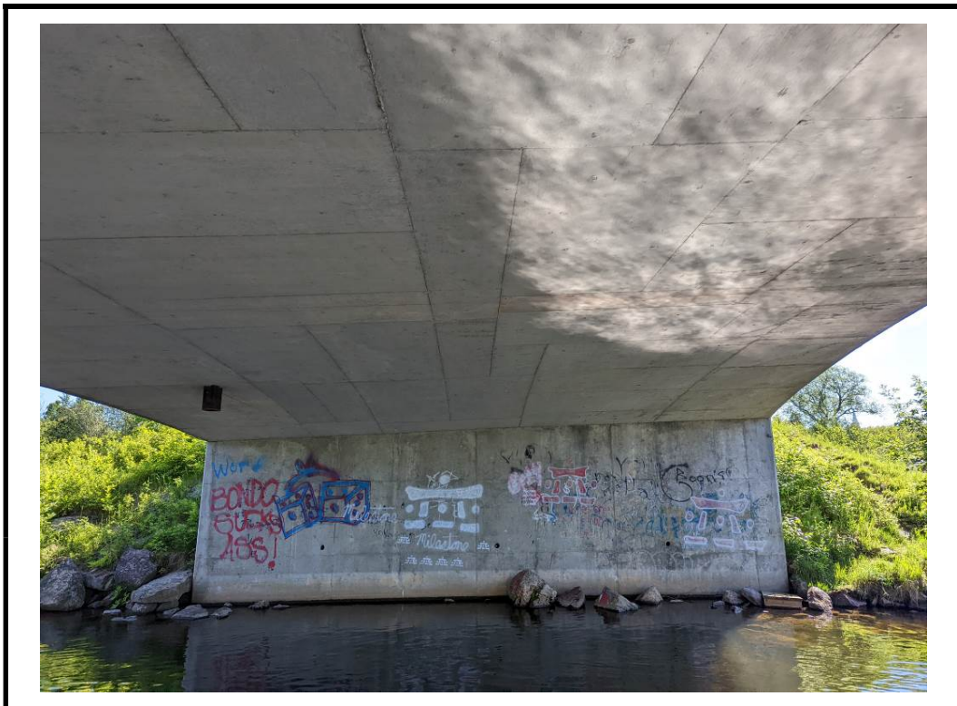
Photo 20 Narrow full length vertical cracks and graffiti noted on abutment walls (Typical)
