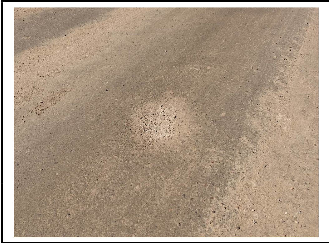
Photo 7 Several small potholes on west approach
