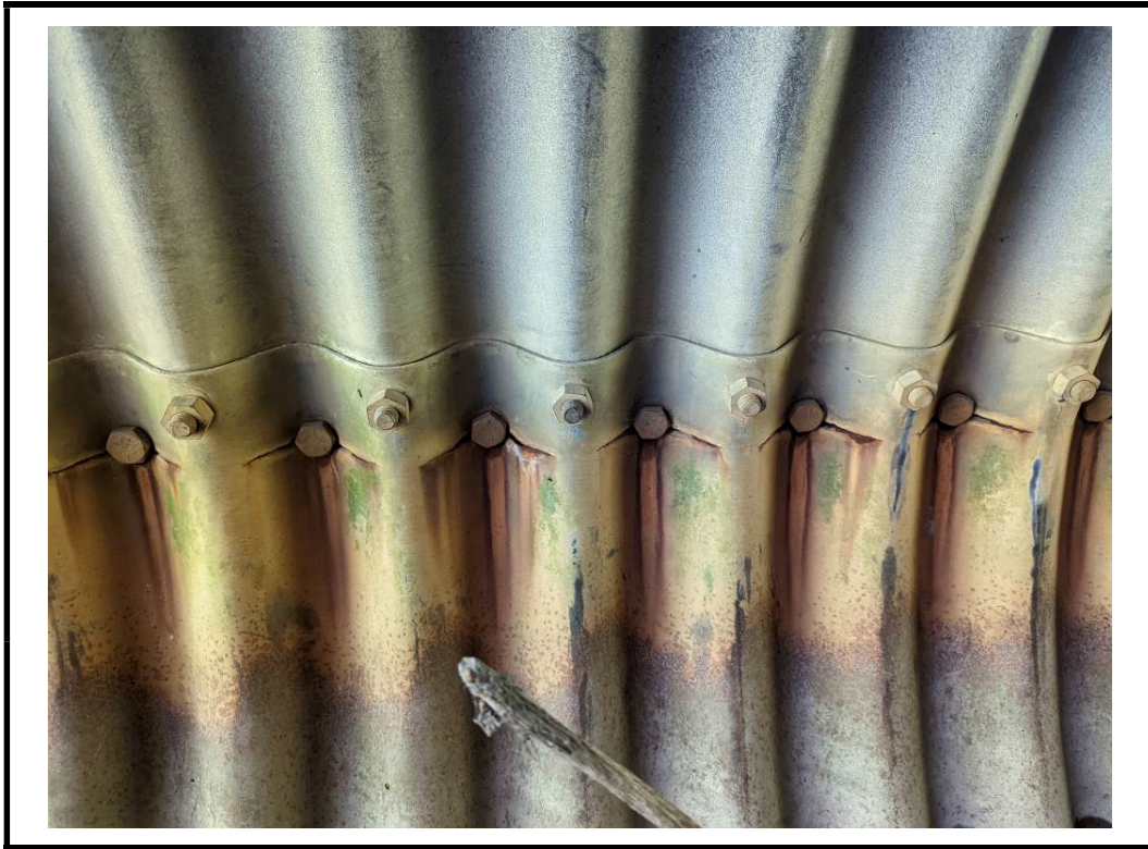
Photo 9 Medium cracking noted along bolt line
