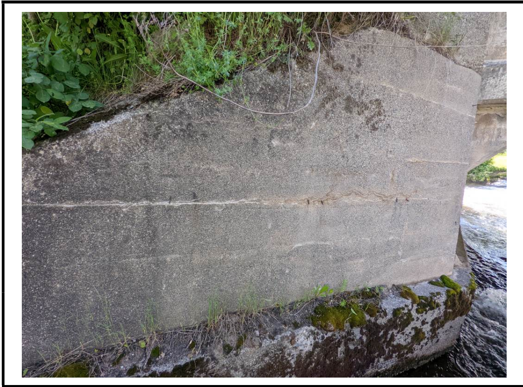
Photo 17 Narrow longitudinal and transverse cracks, damp stains and moos grown at wingwalls (Typical)
