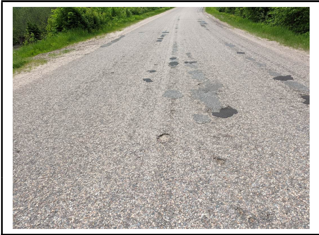
Photo 7 Previous patches, moderate raveling and potholes forming at west approach
