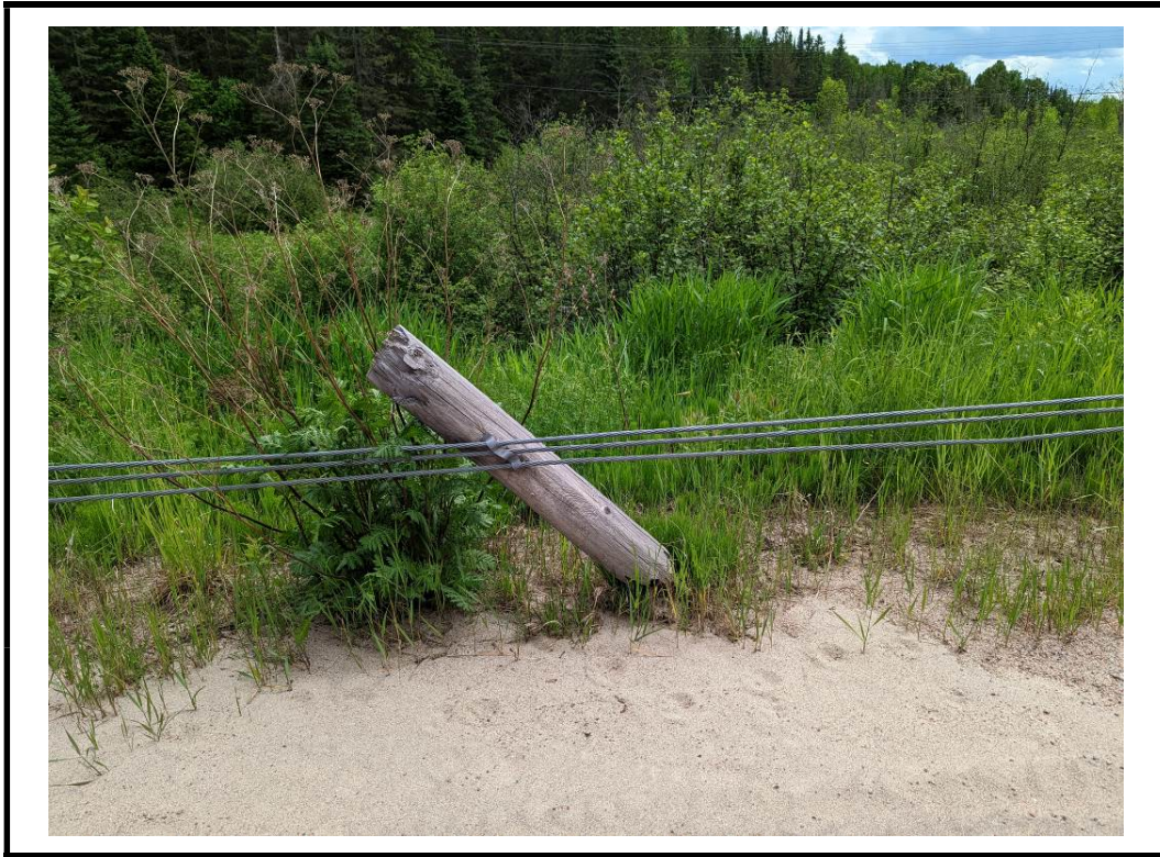
Photo 7 Broken post observed in north barrier
